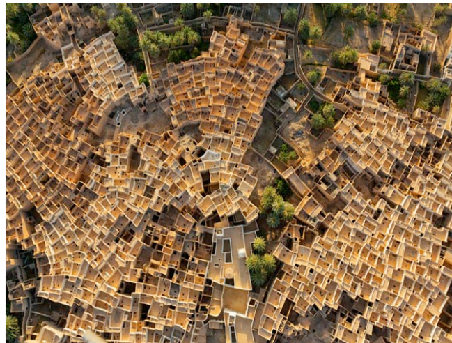
Figure (3. 10) the old city of Ghadames. Source, (Photographer Georg Steinmetz Biography- National Geographic-2013)
