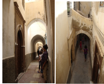
Figure (3. 4) the external facade on the narrow covered street
